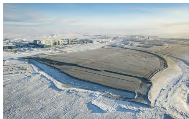
Recognized as one of the best practices in the industry, filtered tailings deposition is used at our Meliadine mine and Pinos Altos complex, and is in the process of being integrated at our LaRonde complex.
